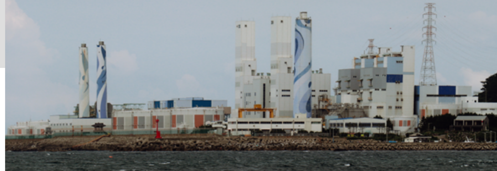
■ Thermal power plant burning palm oil-based bio-heavy oil in Jeju, S. Korea ©Jeju KFEM
